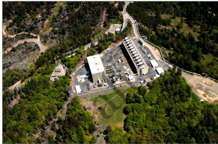
Photo 17-1, Cal Pine Generating Station at the Geysers
